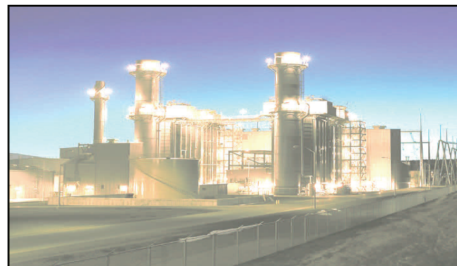
Pacific Klamath Energy Cogeneration Facility
